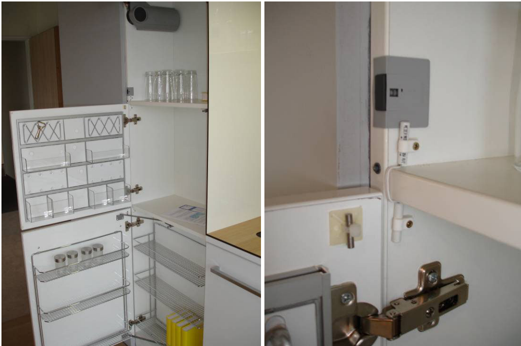
Figure 7: (a) Sensors in the cabinet door (b) Detailed view
