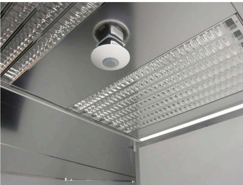
Integration of PIR and door contact sensors into the system. Monitoring of PIR signals onto a tablet PC. Gaining PIR data onto the cloud. Testing sensitivity of PIR sensors and lag time in data acquisition.
