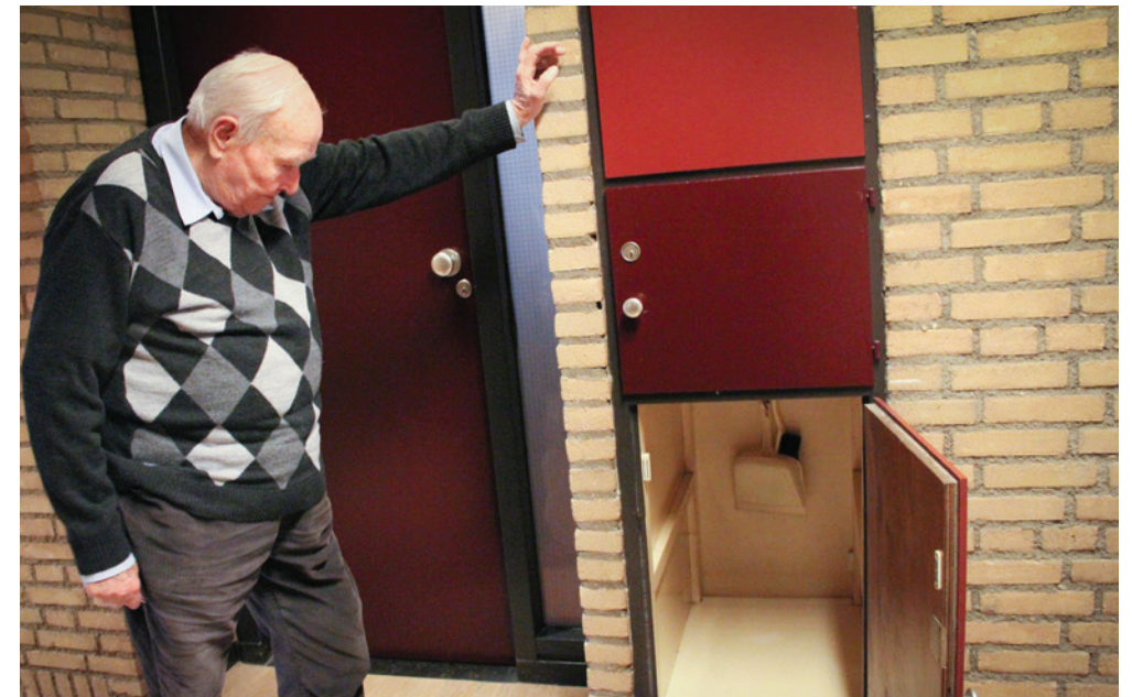
Way in of the kitchen cabinet from the outside
